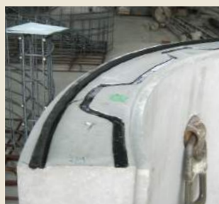
During TS SEAL Lamination
