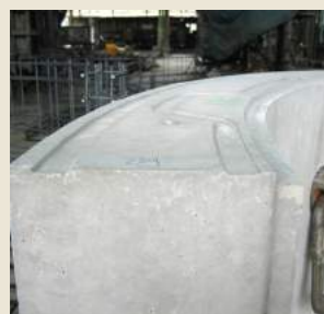
Joint: Before TS SEAL laminated
